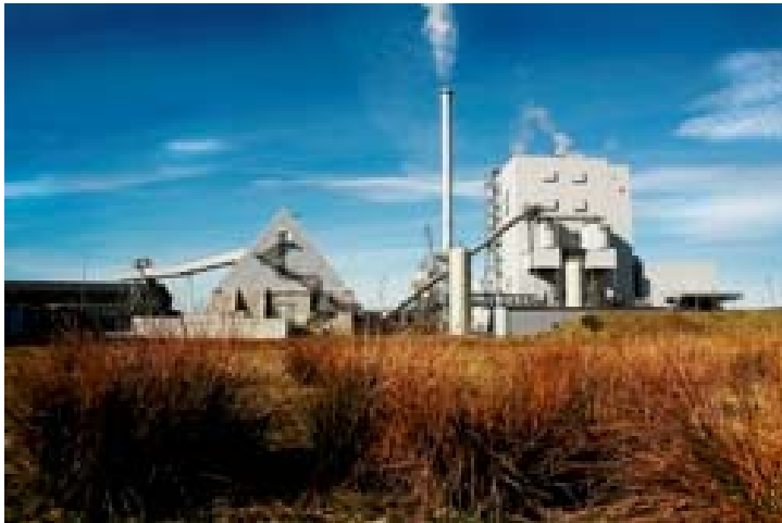
Stevens Croft Plant, Lockerbie
