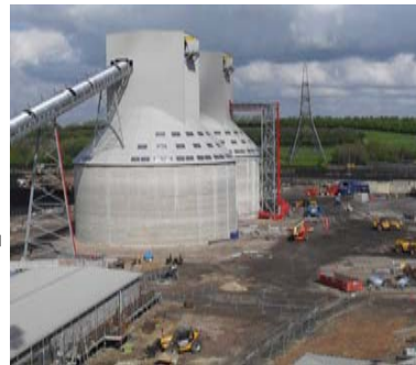
Storage/ Site Processing
